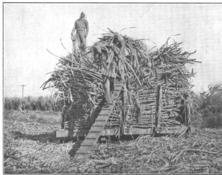
LOADING CARS ON THE TEMPORARY TRACK.
