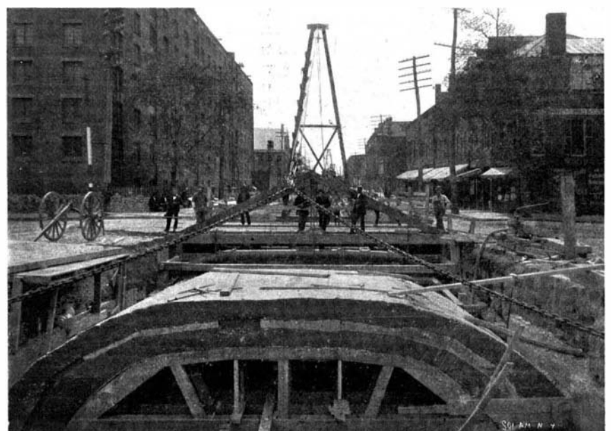
THE MONOLITHIC, CONCRETE, ROOF OF THE TUNNEL.
