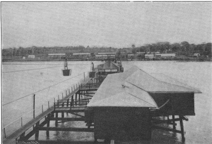
VIEW FROM OFFICE, LOOKING TOWARD PITCH LAKE.
