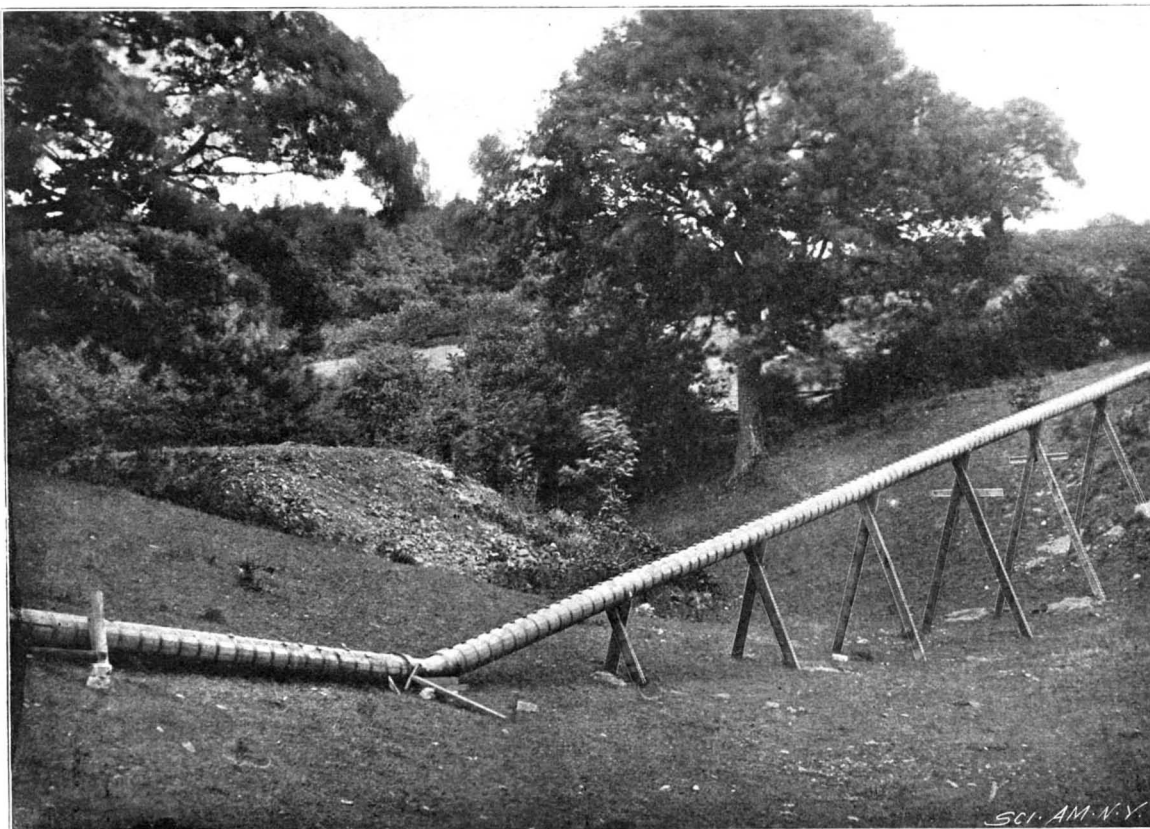
WOOD-PIPING—COMPLETED SECTION ACROSS A VALLEY.
