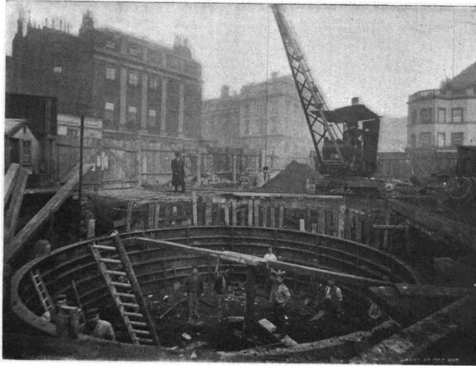
Sinking a Caisson, Preparatory to Excavating the Tunnel.
