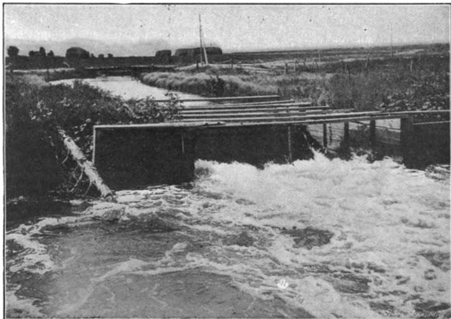
LARIMER AND WELD DITCH, DRAWING WATER FROM ITS TERRY LAKE RESERVOIR AND DELIVERING IT INTO ITS MAIN DITCH.
