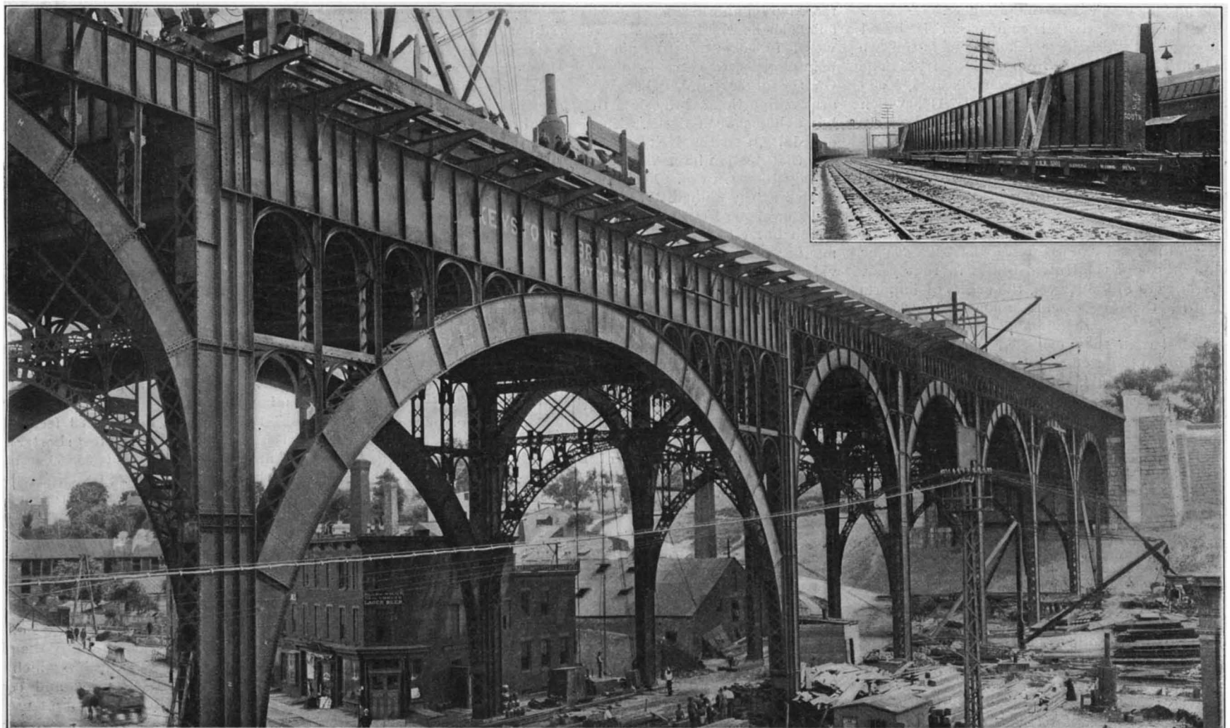
The 130-Foot Arch Across Manhattan Street. RIVERSIDE DRIVE VIADUCT, NEW YORK.—[See page 38.]
