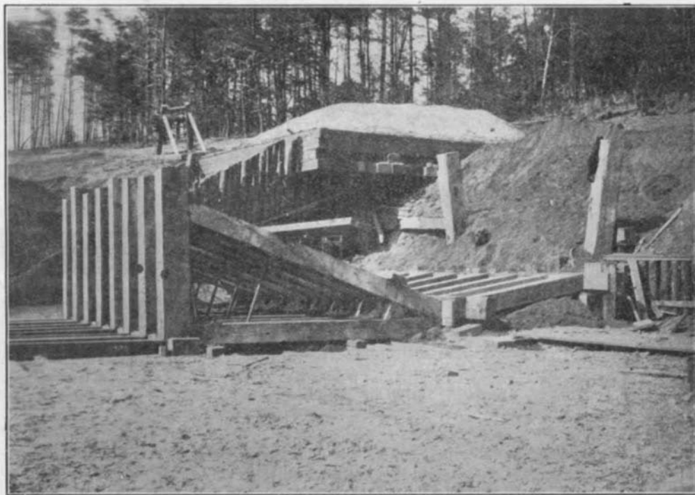
INDIAN HEAD PROVING GROUND—THE BUTTS, SHOWING METHOD OF SUPPORTING PLATE AND BACKING
