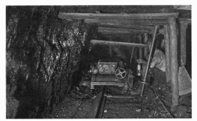
Electric Coal-Mining Machine at Work.
