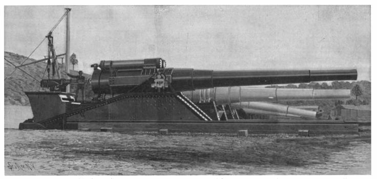
New Navy 12-inch Gun at Indian Head-Muzzle velocity, 2,854 foot-seconds; muzzle energy, 47,994 foot-tons; foot-tons of energy per ton of gun, 893; powder pressure, 16.5 tons per square inch. THE MOST POWERFUL 12-INCH, 40-CALIBER GUN IN EXISTENCE.
