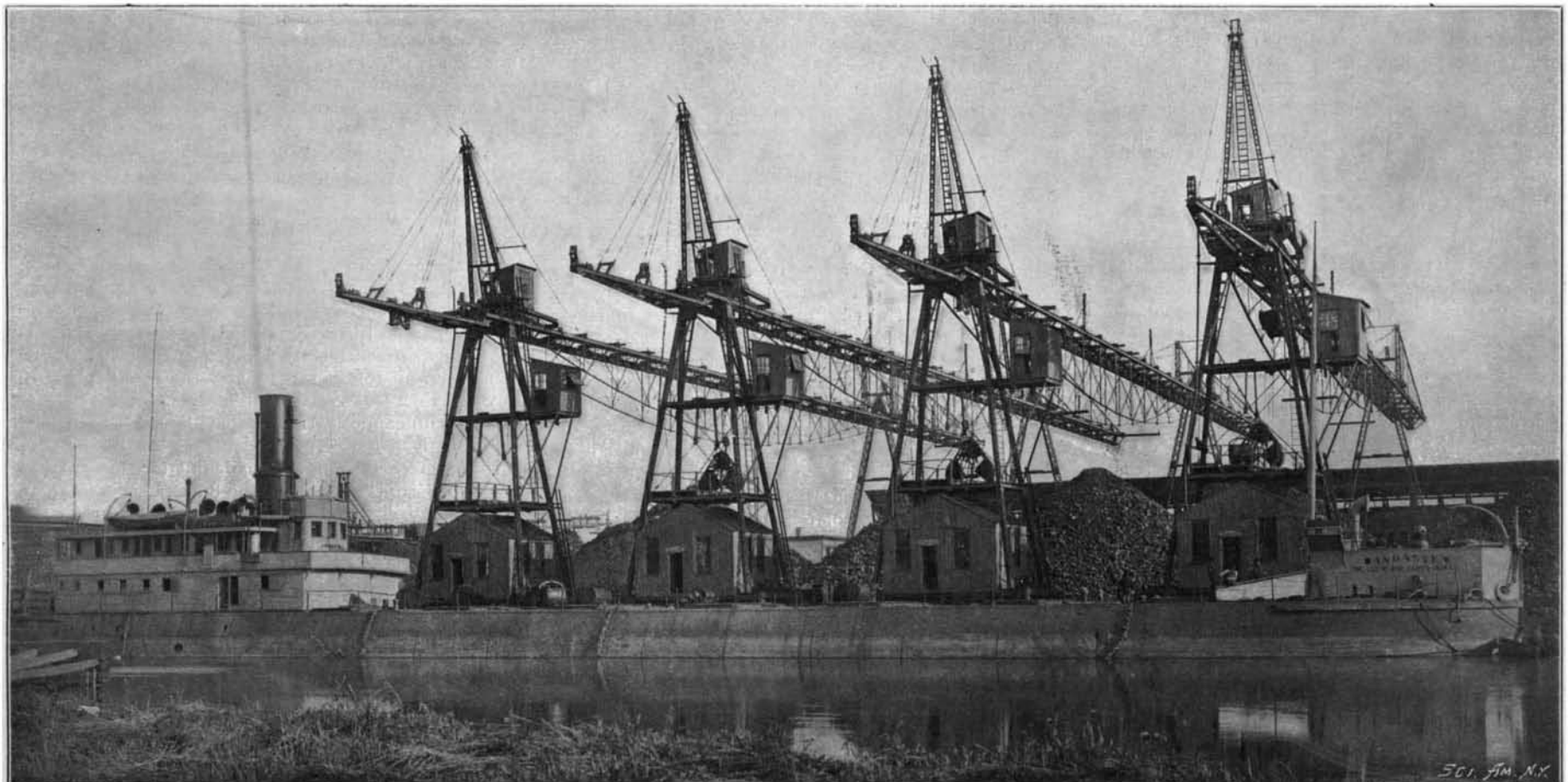
Four-Bridge, Coal Frameway for Unloading Anthracite. HANDLING ANTHRACITE COAL.—[See page 841.]
