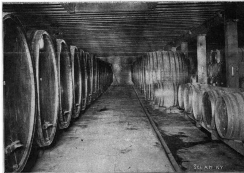
LARGE WINE VATS WHICH WERE USED TO SUPPLY THE FIRE PUMP.
