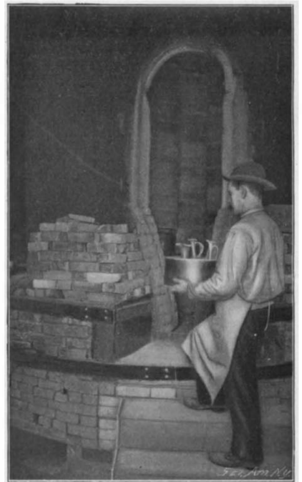
PLACING WORK IN THE KILN.
