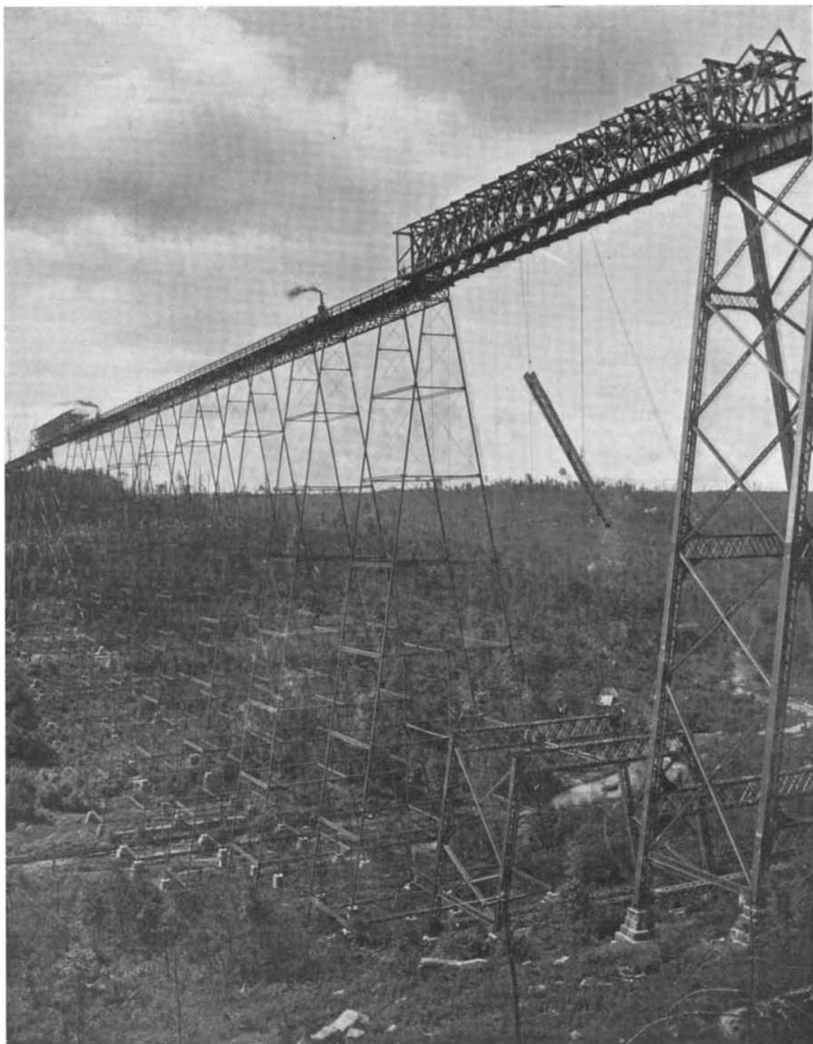
Lowering a Column Section into Position.
