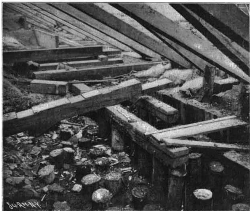
Pile Foundation for Concrete Monolith.
