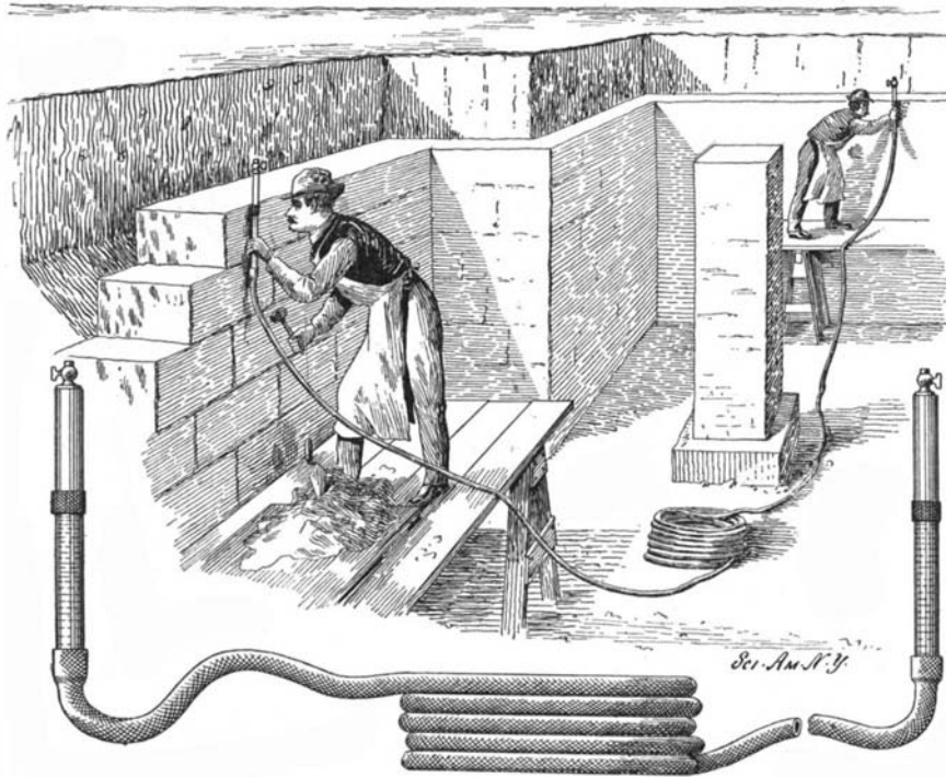
A SIMPLE HYDROSTATIC LEVEL.
