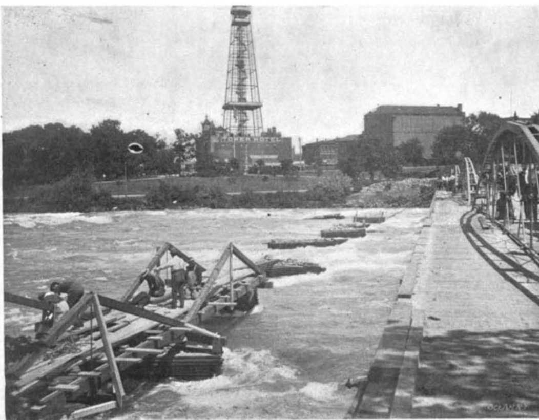
BUILDING A TEMPORARY BRIDGE TO GOAT ISLAND.
