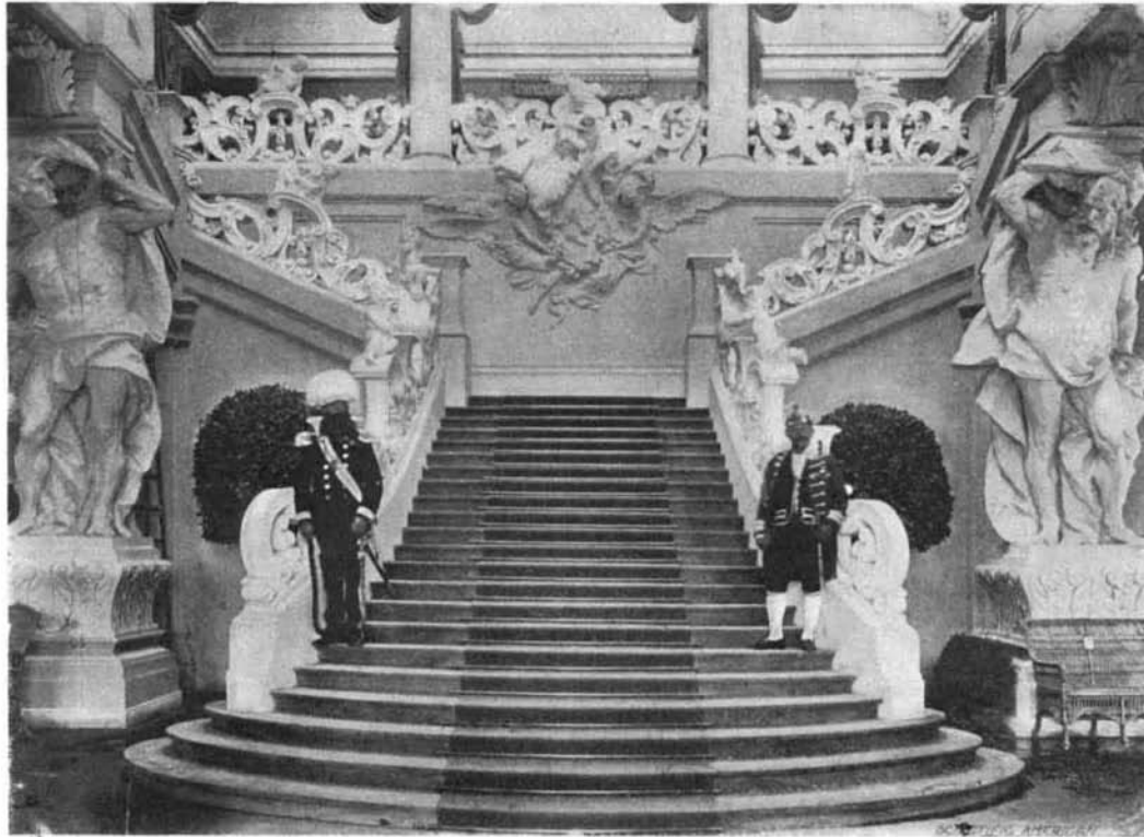
GRAND STAIRCASE, PALACE OF AUSTRIA, AT THE PARIS EXPOSITION.
