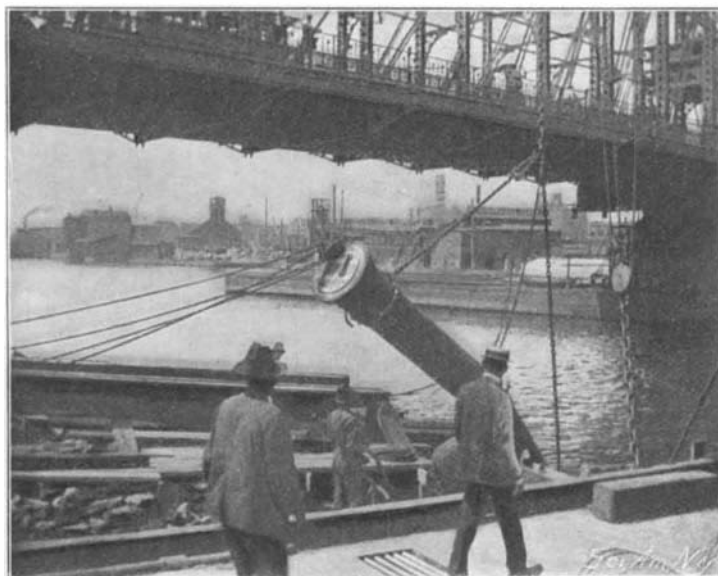
THE LAST LENGTH OF PIPE BEING LOWERED TO POSITION.
