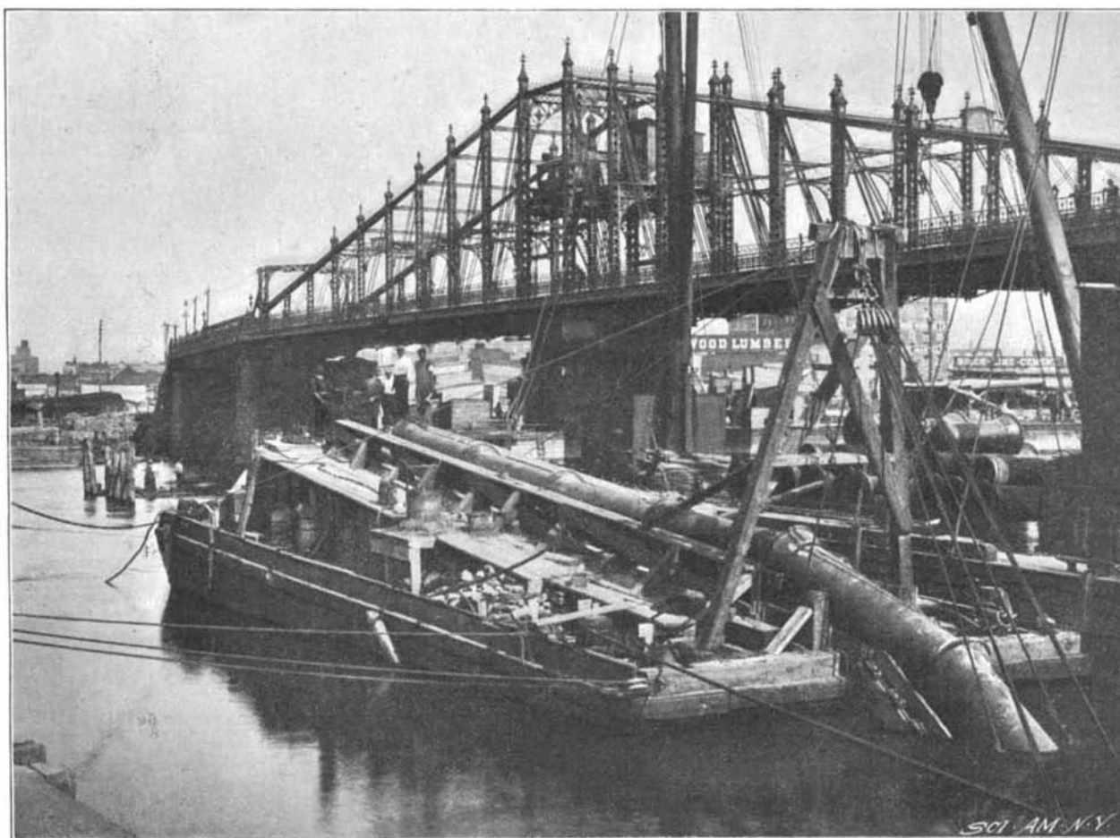
METHOD OF JOINING AND LAUNCHING THE FINISHED PIPE.
