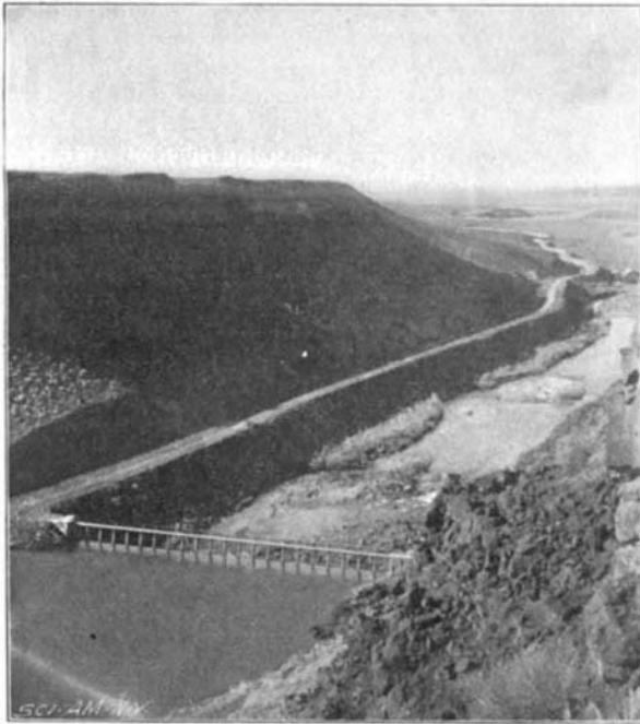
BRUNEAU DAM AND CANAL.
