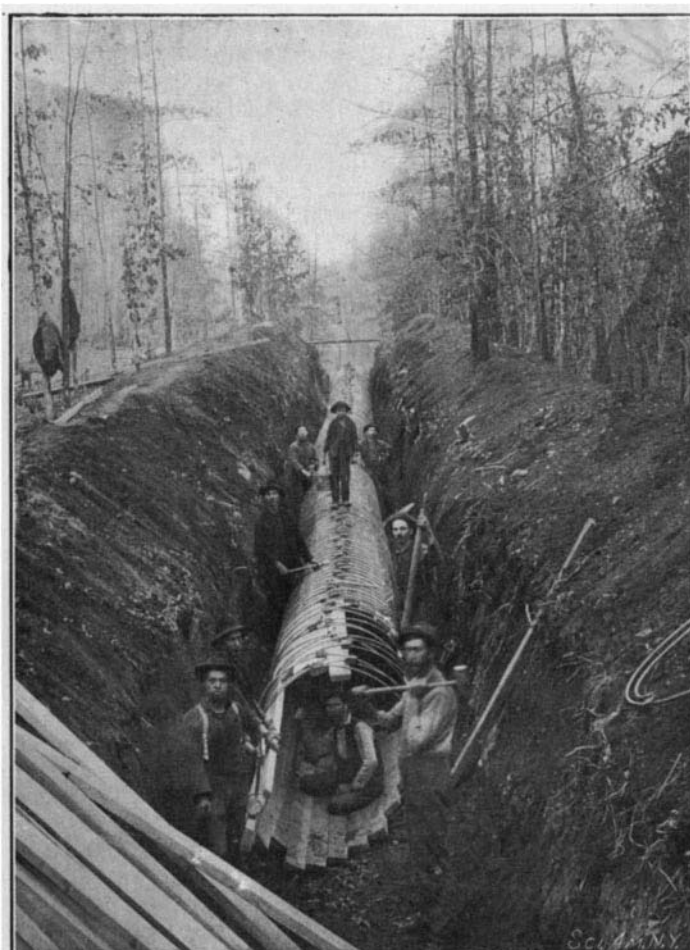
REPAIRING 44-INCH WOODEN PIPE IN THE HAND DITCH.
