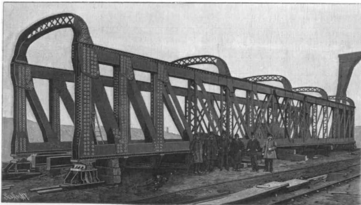
FIRST SPAN OF NEW BRIDGE ACROSS THE TUGELA, NATAL—BUILT IN NINETEEN DAYS.
