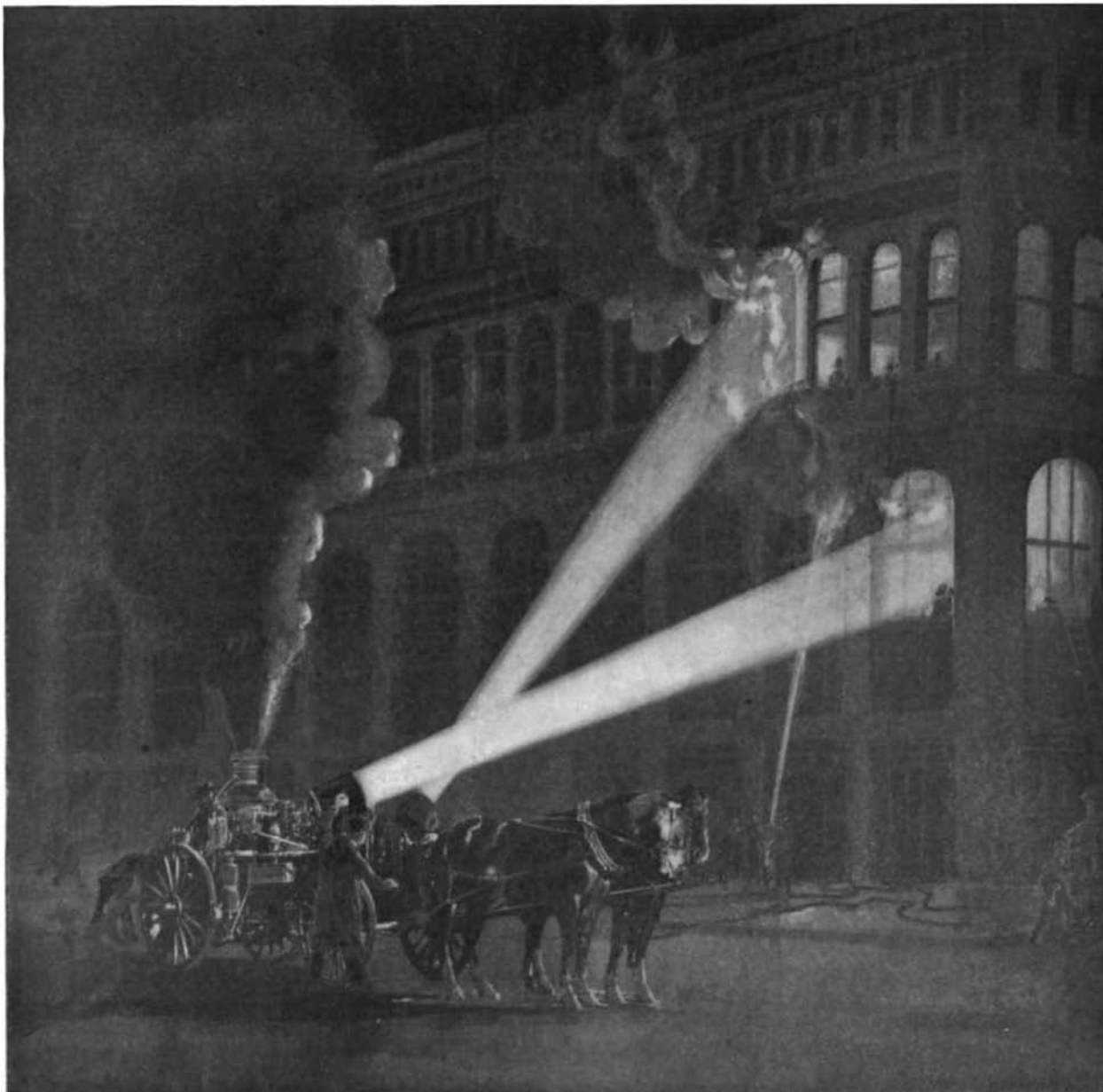
NEW YORK'S LATEST FIRE FIGHTER—THE PORTABLE SEARCH-LIGHT PLANT AT WORK.
