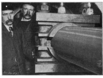
PROPELLER SHAFT REPAIRED AT SEA WITH TWO SPARE CRANK-PIN BRASSES, AND TWO CAPS AND HOLDING-DOWN BOLTS FROM THE MAIN ENGINE.
