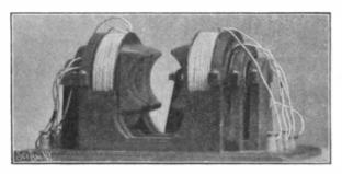
SINGLE CIRCUIT, BIPOLAR ELECTRO-MAGNETIC MACHINE.
