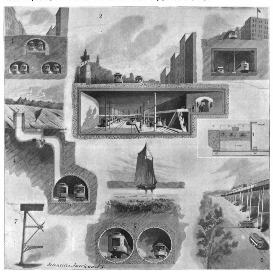
1. The four-track road in two tunnels below the Park Avenue tunnel. tunnels beneath Harlem River. 2. Fourteenth Street station, looking north. 3. Two-track line below Lenox Avenue. 4. Ventilating shaft for tunnel beneath Central Park. 5. Tubular tunnels beneath Harlem River. 6. Elevated portion at One Hundred and Twenty-fifth Street. 7. Details of viaduct construction. 8. Details of track.
