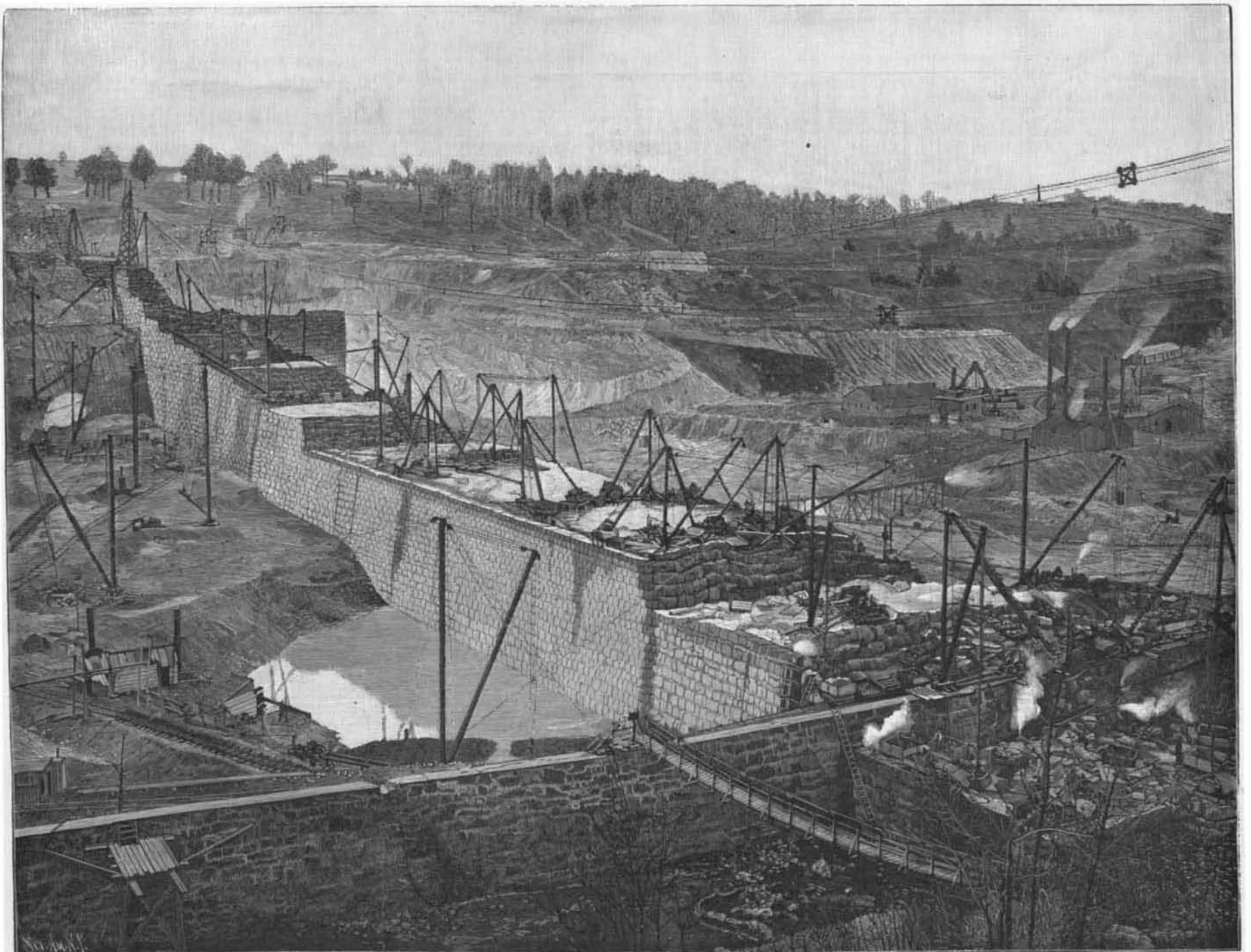
Fig. 2.—Up-stream Face of Dam; Bed of Reservoir will be at Present Level of Masonry at Center of Dam. THE GREAT CROTON DAM—NEW YORK CITY'S WATER SUPPLY.—[See page 86.]
