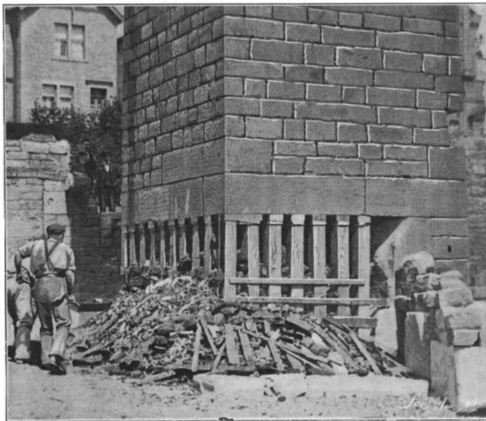
BASE OF THE STACK UNDERPINNED, AND FUEL LAID READY FOR BURNING.
