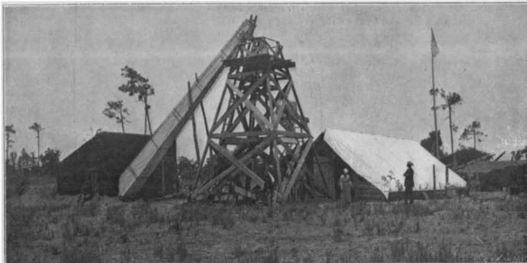
The 40-foot Photo-Heliograph on its Scaffold.
