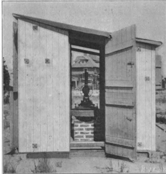
Portable Transit House which has been used on Many Eclipse Expeditions.
