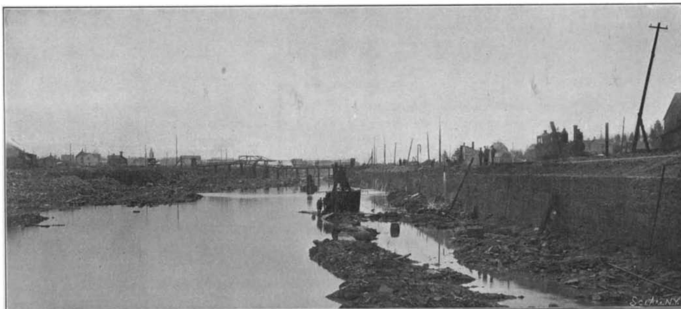
Width on bottom, 200 feet; depth, 23 feet; length, 1¼ miles; available head, 18 feet.
