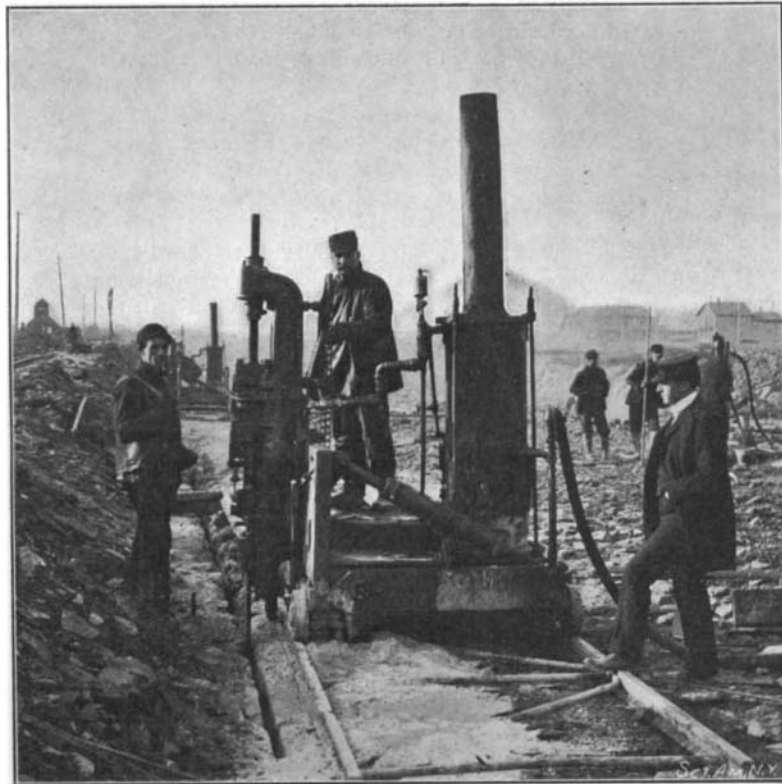
CHANNELING-MACHINES AT WORK IN ROCK CUT.
