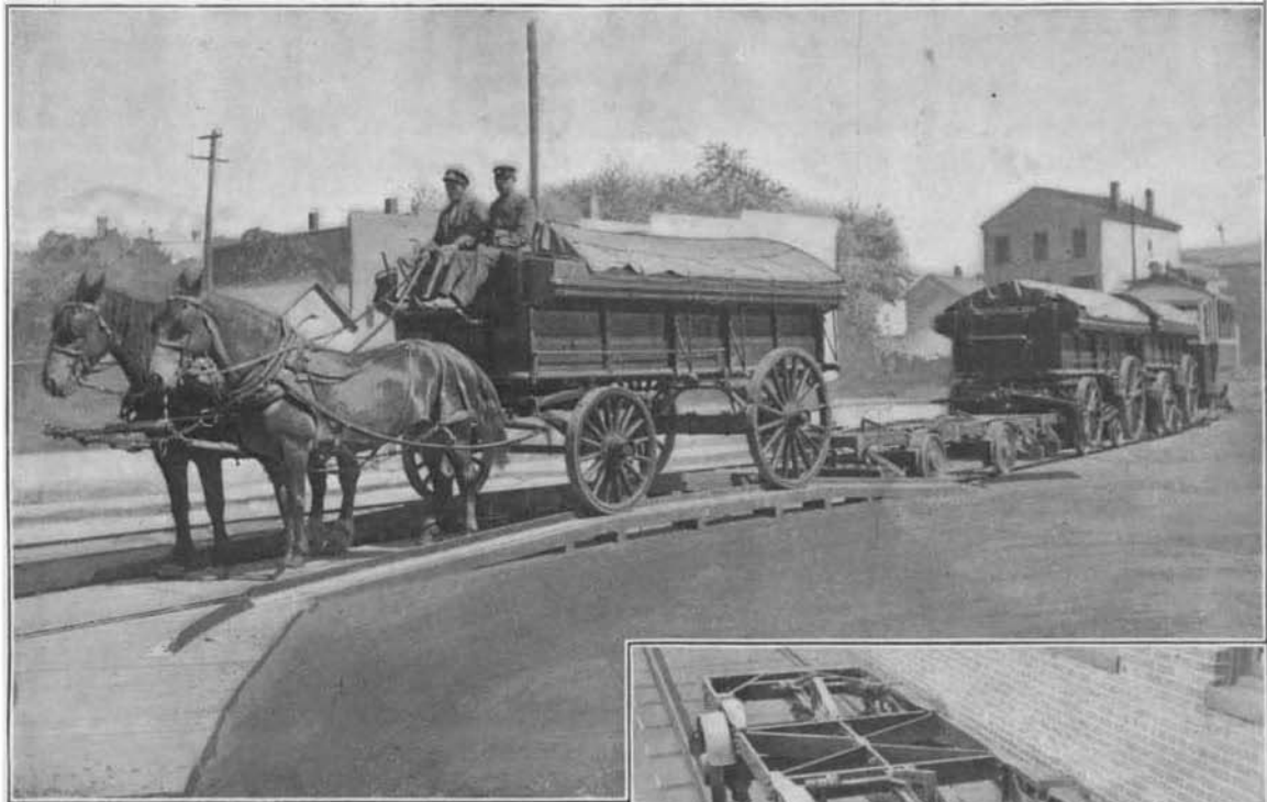
1.—RAIL WAGON HAULED UP INCLINED PLANE, CLEAR OF TRUCK.
