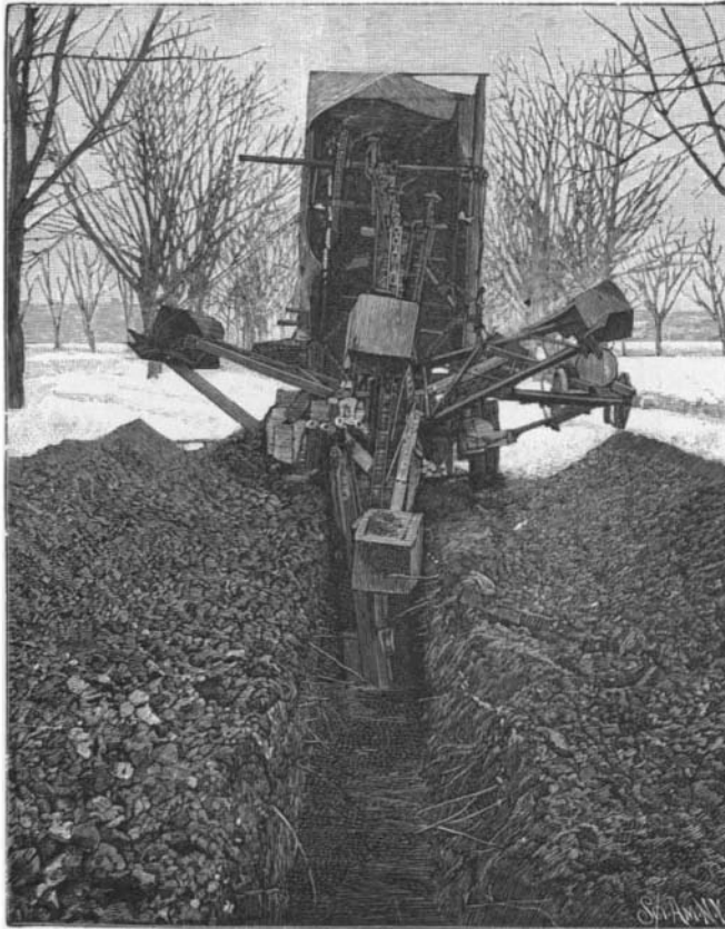
END VIEW SHOWING TRENCH AND SPOIL BANKS.
