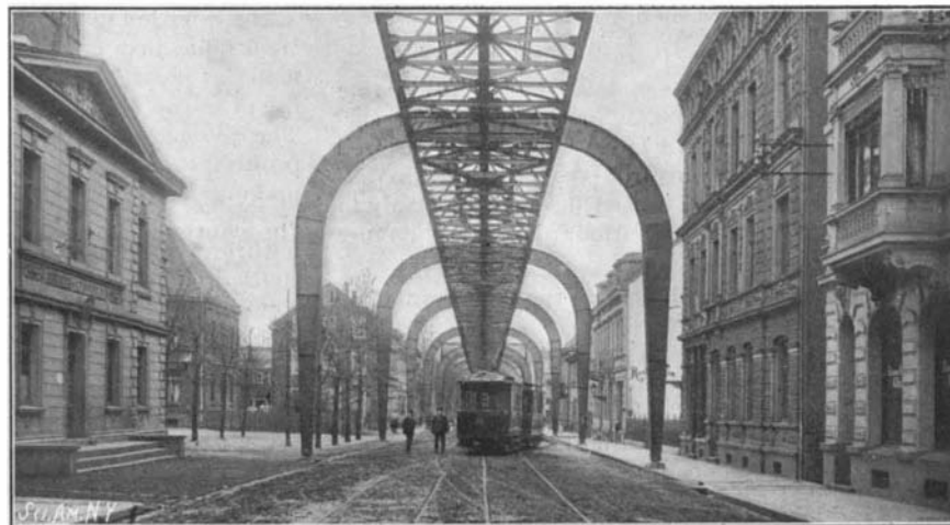
THE INVERTED U-FRAME PIERS USED ON SUBURBAN STREETS AND HIGHWAYS.
