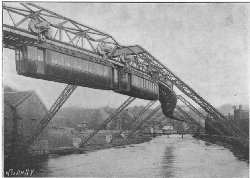
A TWO-CAR TRAIN ON THE LANGEN SINGLE-RAIL SUSPENDED RAILWAY ABOVE THE WUPPER RIVER.
