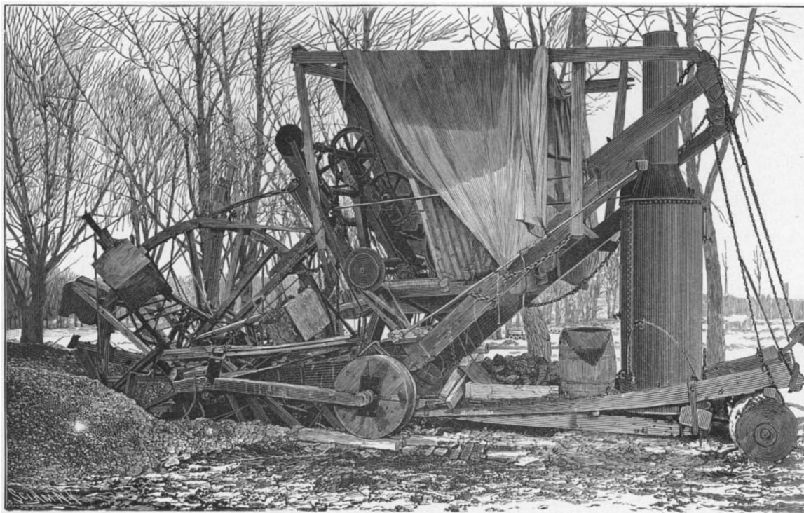
MACHINE FOR TRENCH AND DITCH EXCAVATION.
