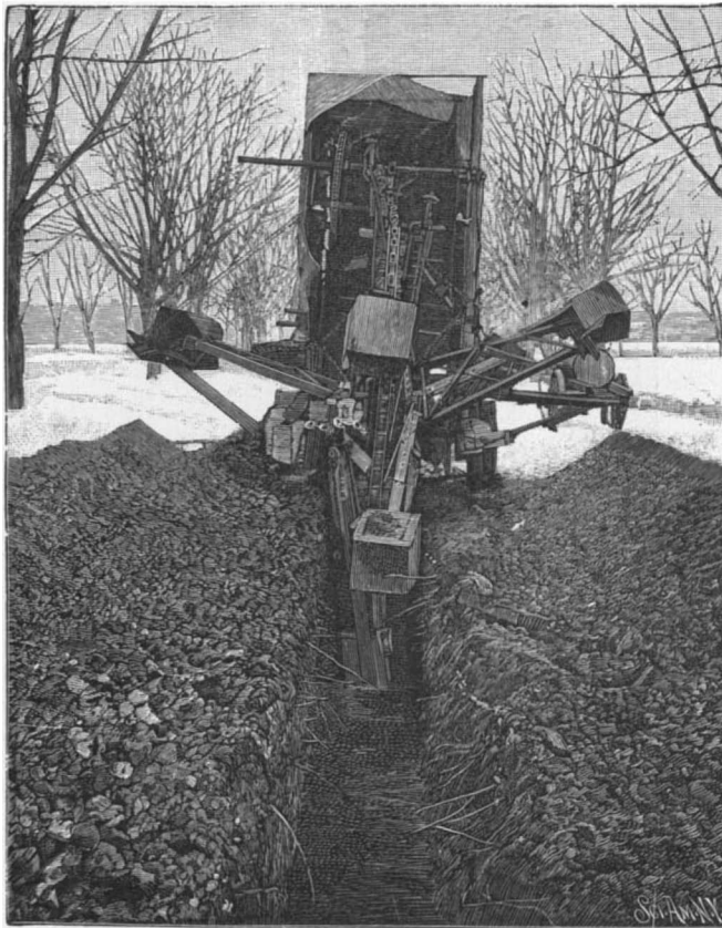
END VIEW SHOWING TRENCH AND SPOIL BANKS.
