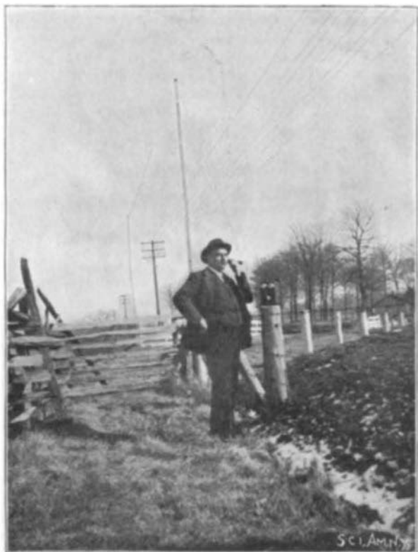
HOME-MADE FENCE TELEPHONE SYSTEM.
