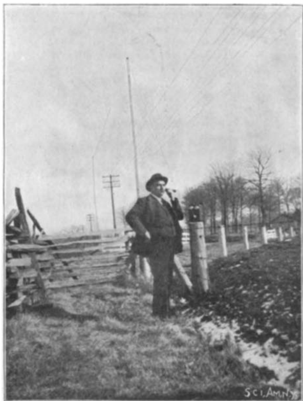
HOME-MADE FENCE TELEPHONE SYSTEM.
