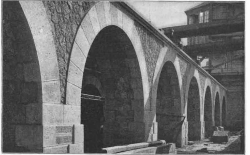
Interior Line of Arches—Masonry Approach.
