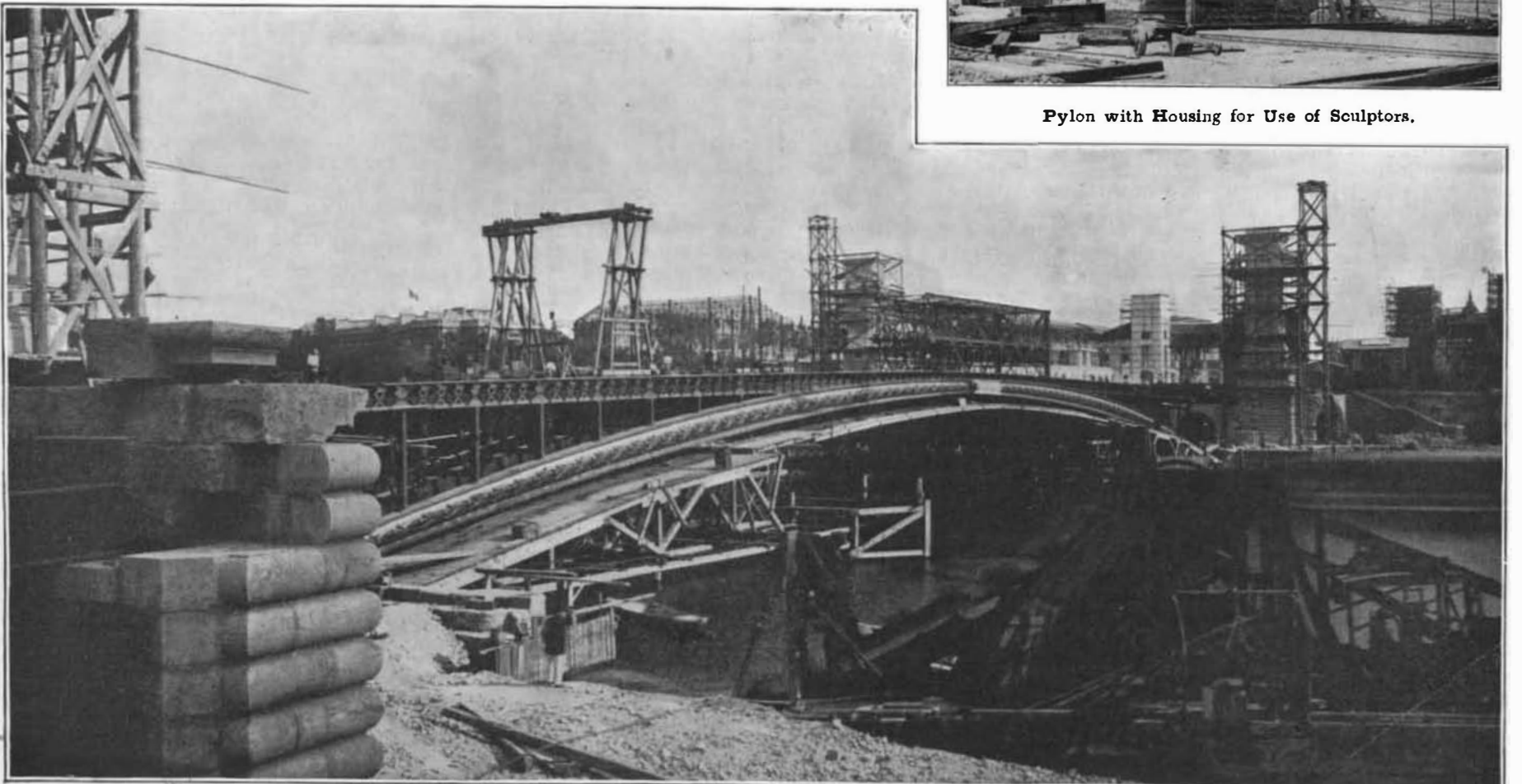
View from Right Bank of Seine During Construction.
