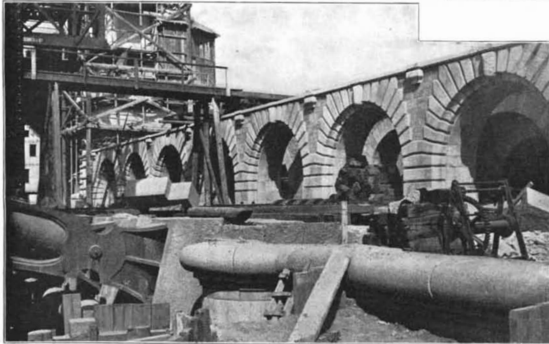
Masonry Approach—Footings of Metallic Arch Shown at Left.
