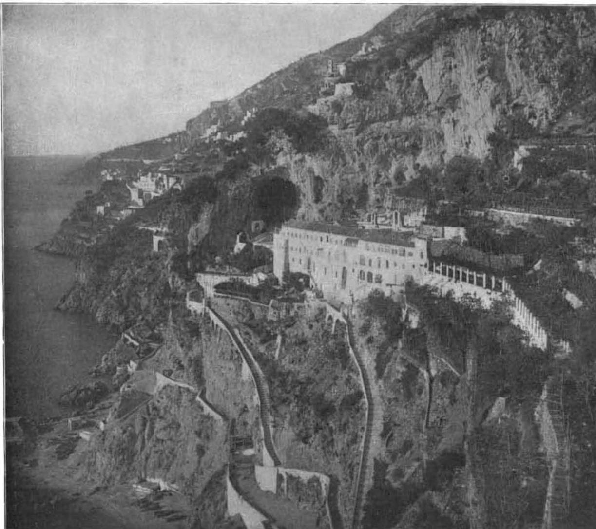
AMALFI—GRAND HOTEL OF THE CAPPUCCINI, RECENTLY DESTROYED BY A LANDSLIDE.
