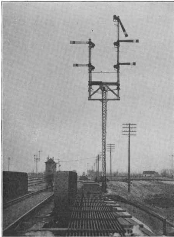
"Home" Signals. Top Blades for Passenger and Bottom Blades for Freight Tracks.
