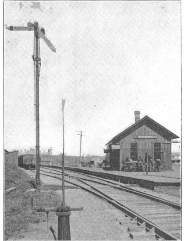
"Advance" Signal, Dropped to Indicate Right Track Clear.
