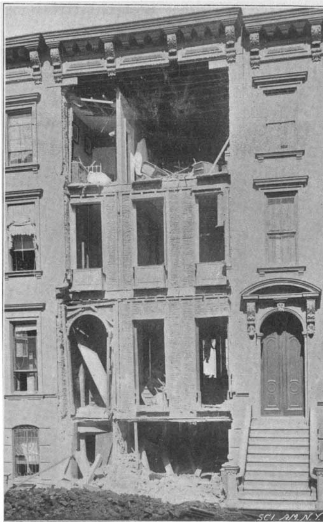
GAS EXPLOSION IN A RESIDENCE IN NEW YORK CITY.
