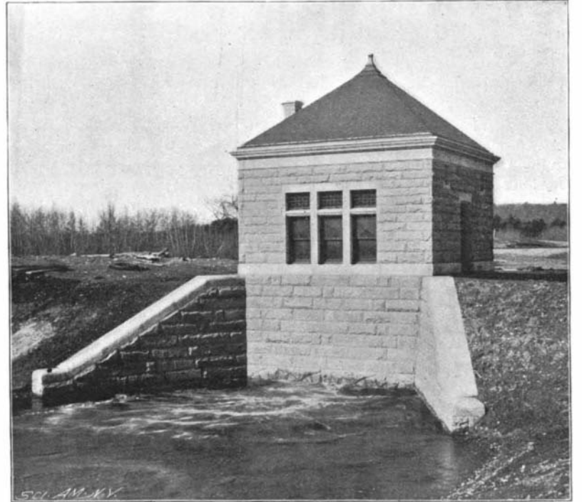
TERMINAL CHAMBER, WACHUSETT AQUEDUCT.
