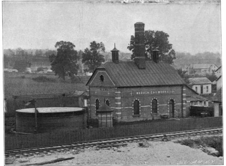
THE WABASH, IND., ACETYLENE GAS PLANT BEFORE THE EXPLOSION.
