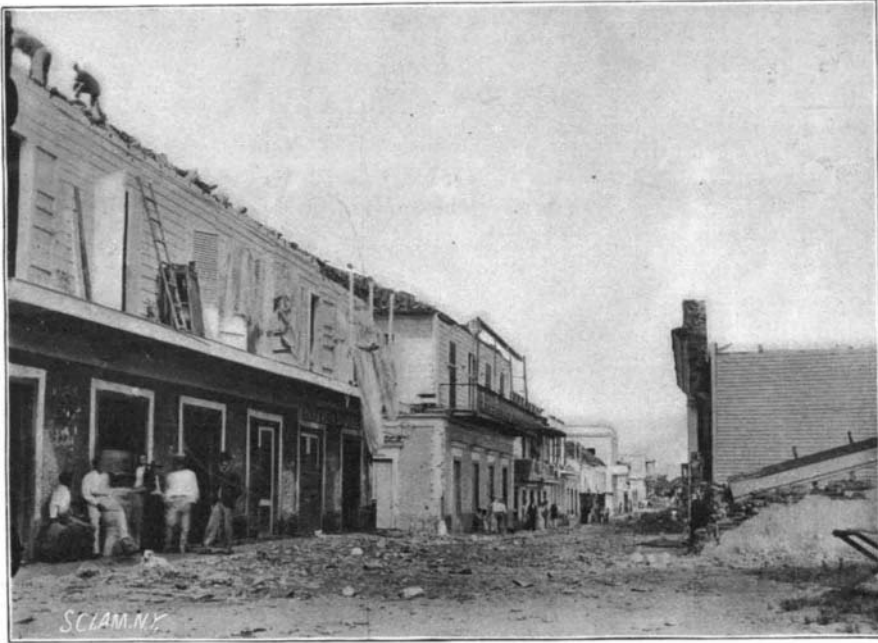
DAMAGE IN THE MAIN STREET OF CAGUAS.
