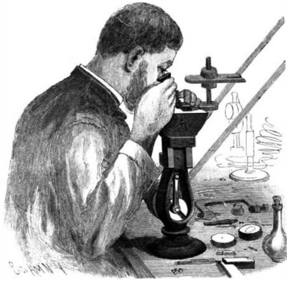
JIG-FILE FOR FINISHING DIES.
