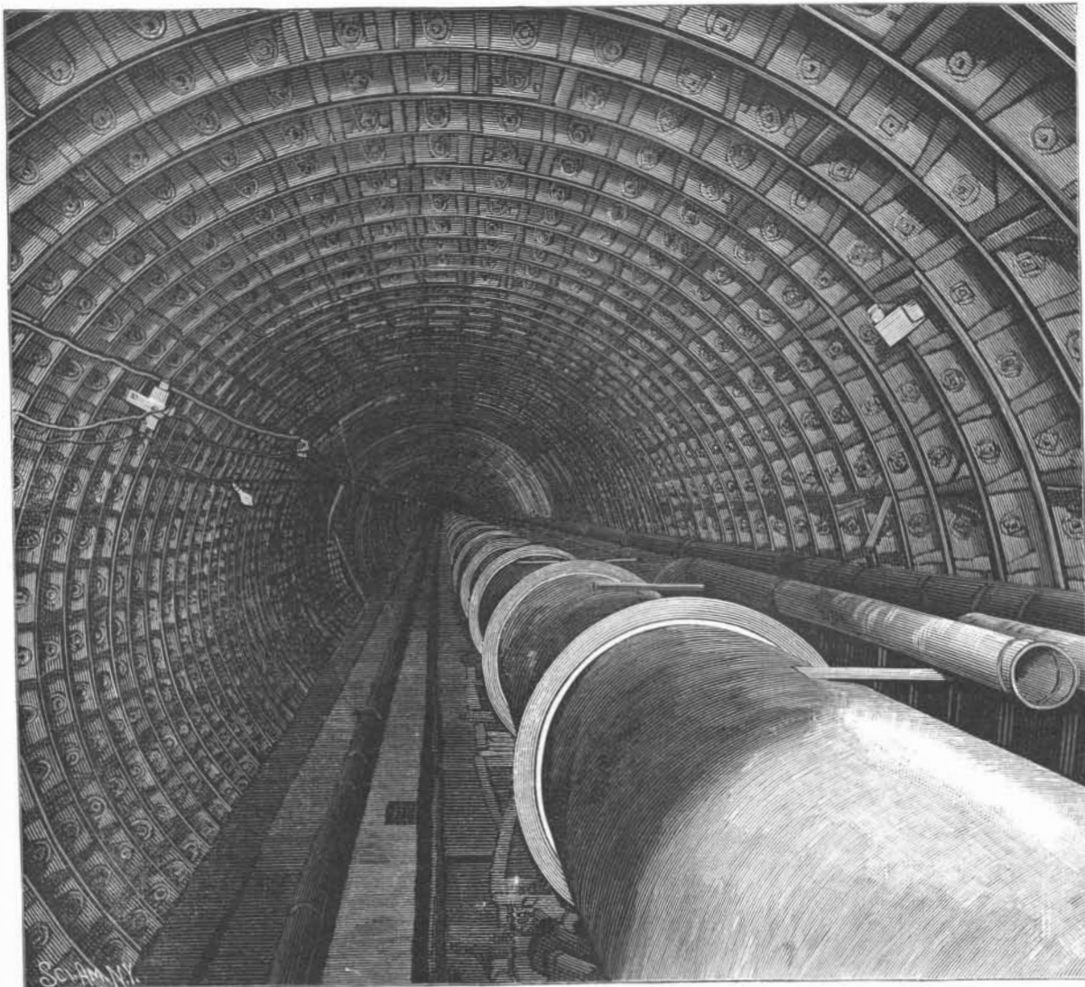
Tunnel for Gas Mains Beneath East River.
