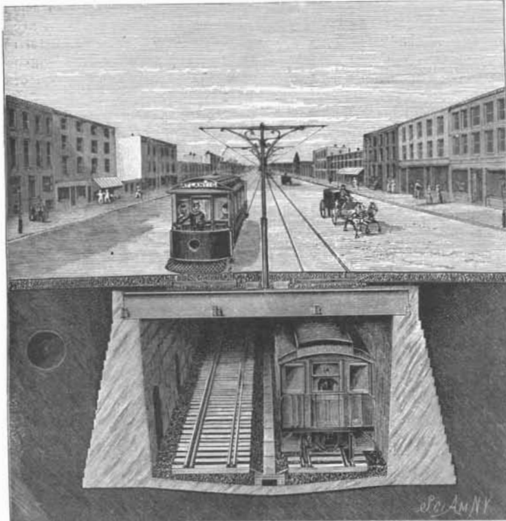
Construction Beneath Atlantic Avenue, Brooklyn.
