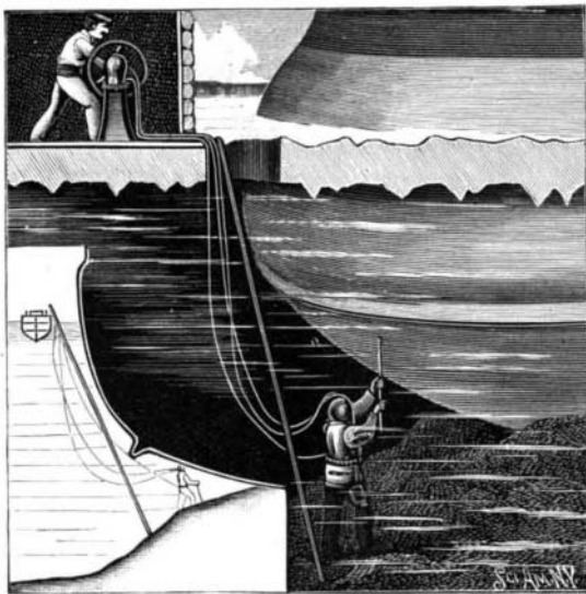
Fig. 1.—OPERATION OF RAISING THE CRUISER "ROSSIA."
