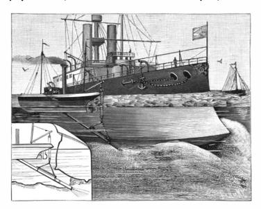
Fig. 2.—DISINTEGRATING THE MUD AND SAND UNDER THE "ROSSIA."
