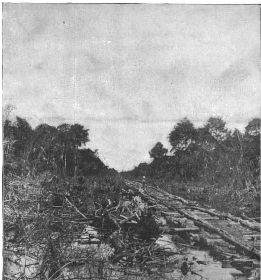
Corduroy Foundations for Railroad Fill Across the Swamp.
