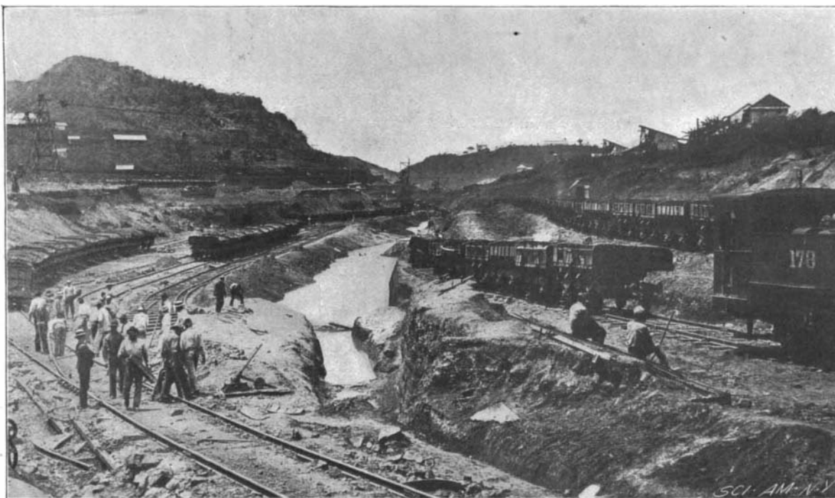
7.—The Work at Outlet of Culebra Cut on Pacific Slope.
