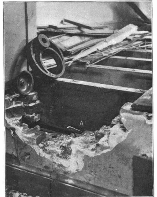
Threshold of Rear Exhibition Room, Showing Concealed Tube, A.
