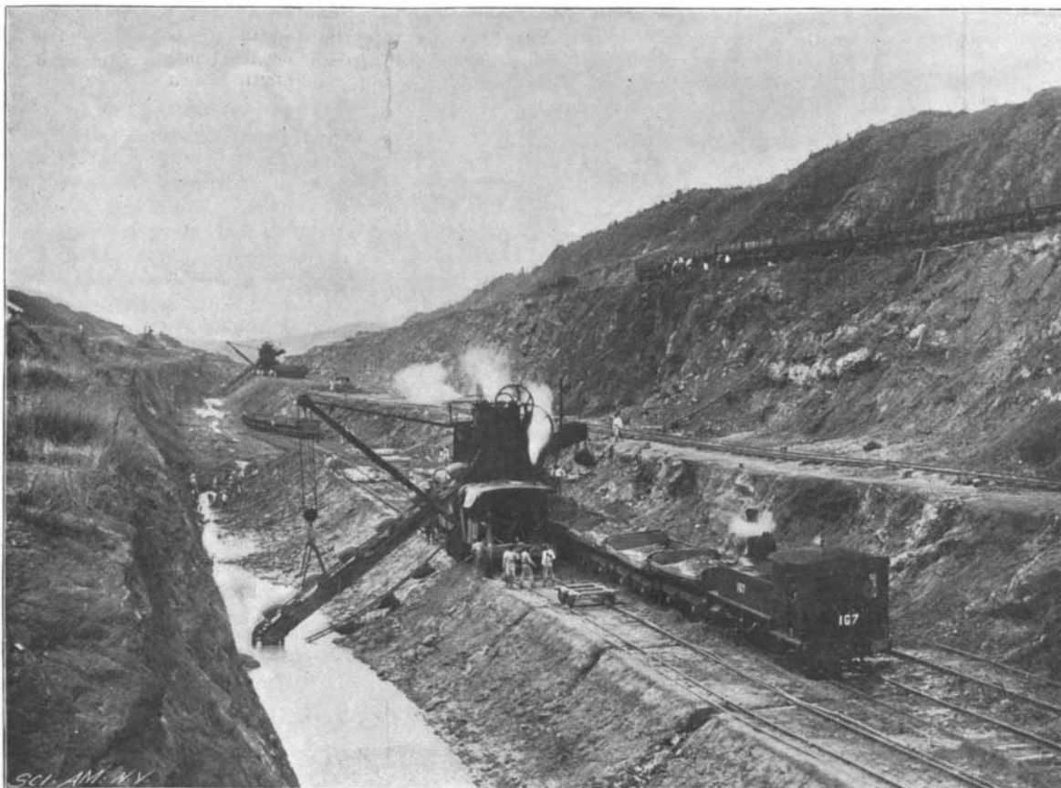
6.—French excavators at Work in the Emperor Cut.
