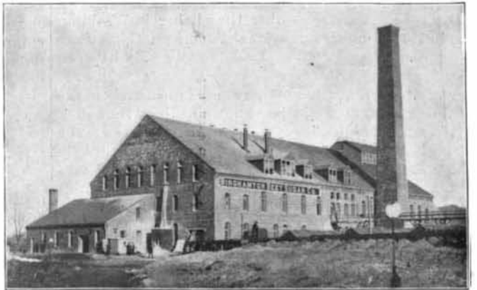
General View of the Exterior of the Building.
