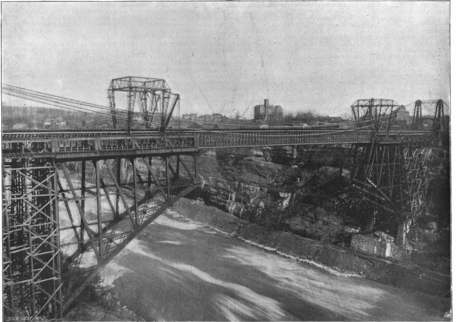
THE BRIDGES OF NIAGARA GORGE—NIAGARA RAILWAY ARCH BRIDGE. SPAN, 550 FEET; RISE, 114 FEET.—[See page 396.]
