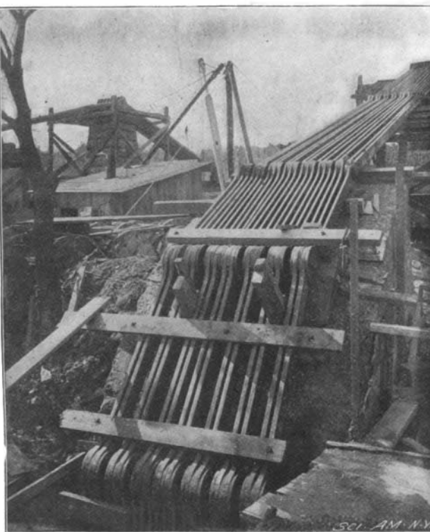
Lewiston Bridge—One of the Anchorages.
