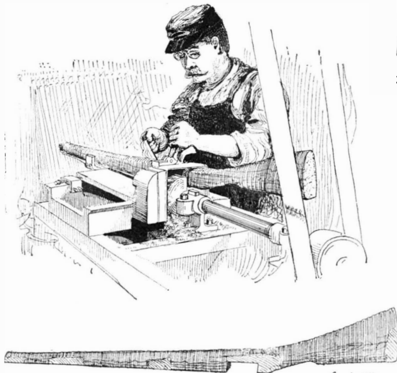
10.—Slotting the Stock—Roughing Cut Preparatory to Bedding.
